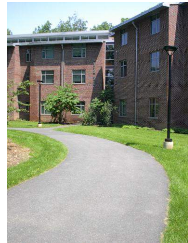
Figure 5.3.1-10. This standard asphalt path is 8 feet wide and includes a stone stormwater bed that is 14 feet wide to support an emergency vehicle. The grassed edges are constructed of reinforced turf grids over the stormwater bed. The bed receives runoff from the roof leaders of the adjacent building.
