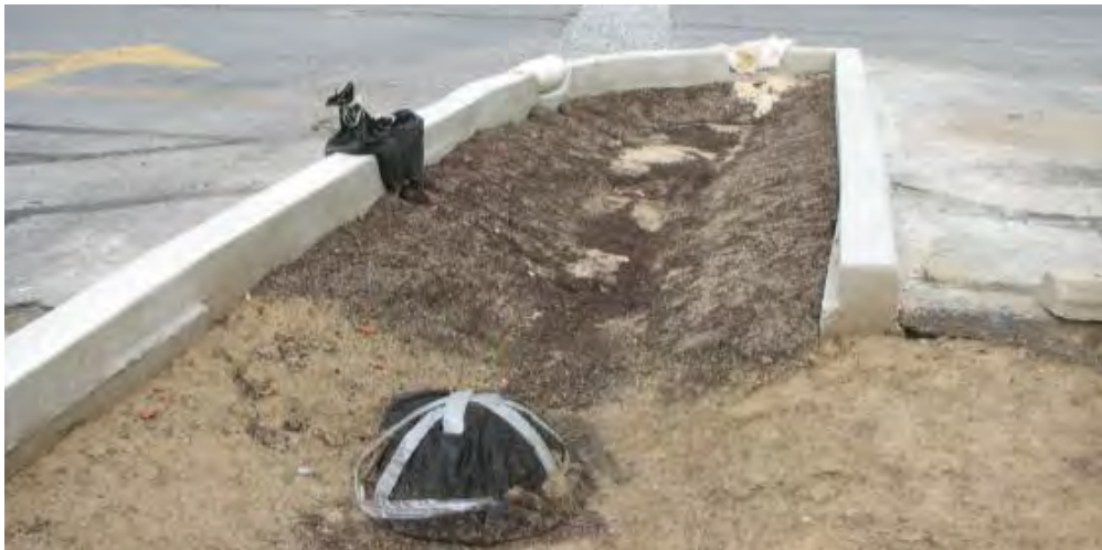
Figure 5.3.4-25. Inlet protection is placed over a domed riser to prevent sediment from entering the system.
