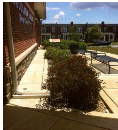
Figure 5.3.11-5. Flow-through stormwater planter boxes adjacent to this library receive roof runoff and provide plantings within the hardscape seating area. Overflow from these planter boxes is directed to a bioretention area (right side of photo). River cobbles (not shown) were added to eliminate any tripping hazard in a high-use area by reducing the depth of the planter box edge to the finished surface.
