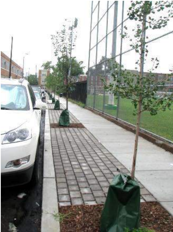
Figure 5.3.3-12. Between the trees in this stormwater tree trench, the soil is extended beneath the porous pavers to provide additional soil volume for the trees.
