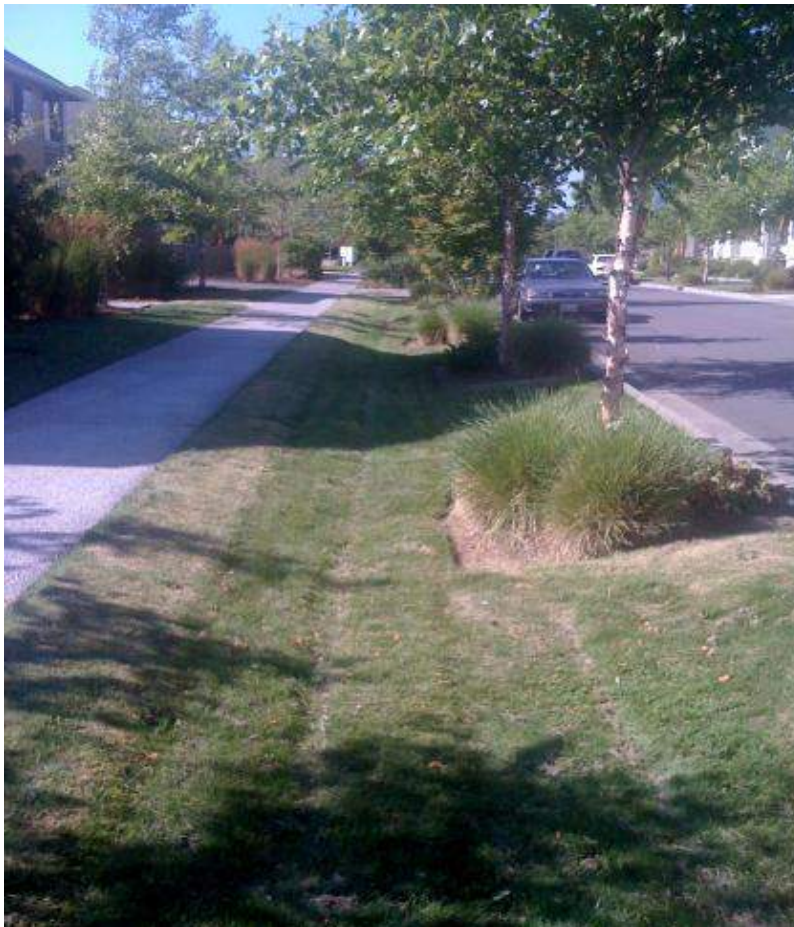
Figure 5.3.5-1. This vegetated swale in a residential area is broad and shallow. Curb cuts allow street runoff to enter the swale.
