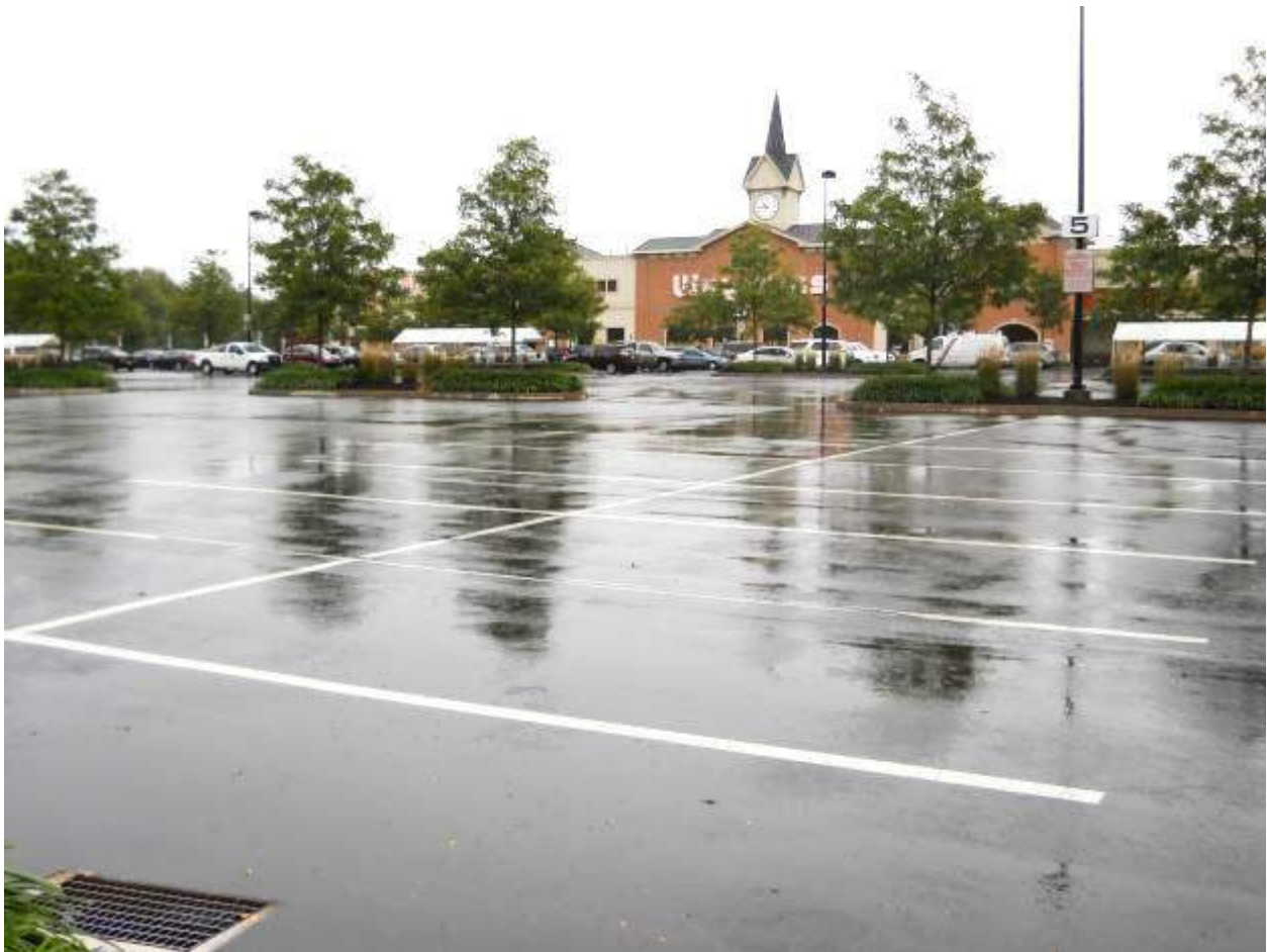
Figure 5.3.2-8. This supermarket parking lot required a level surface. Infiltration beds were placed at the native soil interface, beneath the fill material and parking lot.
