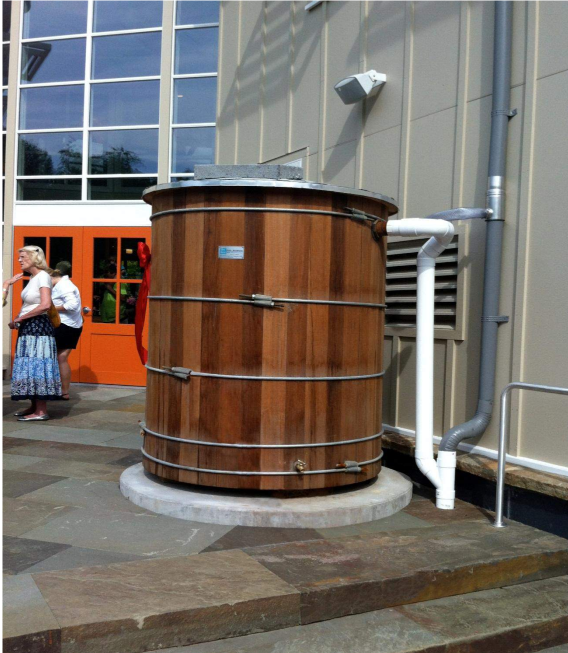
Figure 5.3.9-5. This wooden cistern captures roof runoff at a research facility. The water is used for both toilet flushing and research needs. The captured runoff was more suitable and required less treatment for research use than the available potable water supply.
