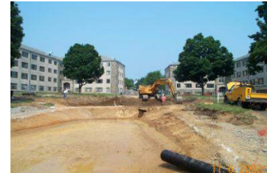
Figure 5.3.1-12. The stormwater bed beneath this pervious concrete plaza was used as a temporary sediment basin (with basin bottom at least 2 feet above final stormwater bed bottom elevation) during construction of the site. After the surrounding site work was completed, the sediment was removed and the bed excavated to its final depth. The stormwater bed and overlying pervious pavement were then installed.
