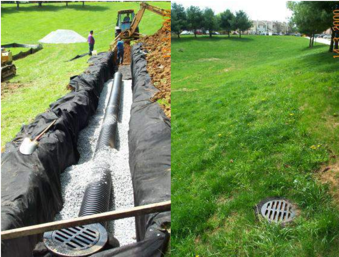
Figures 5.3.3-1a and b. Infiltration trench during installation and afterwards.
