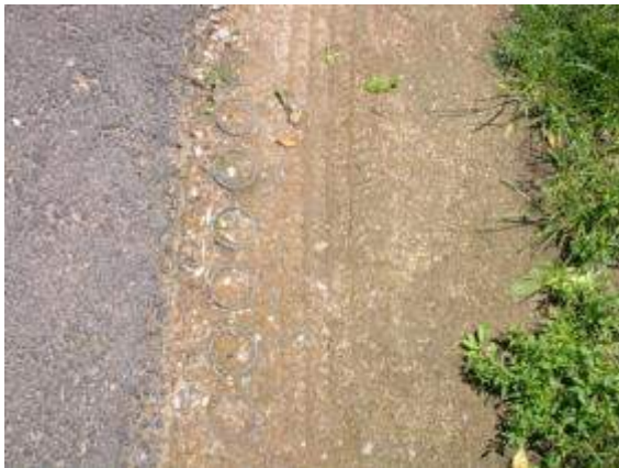
Figure 5.3.1-7-e. Reinforced Turf or Gravel
