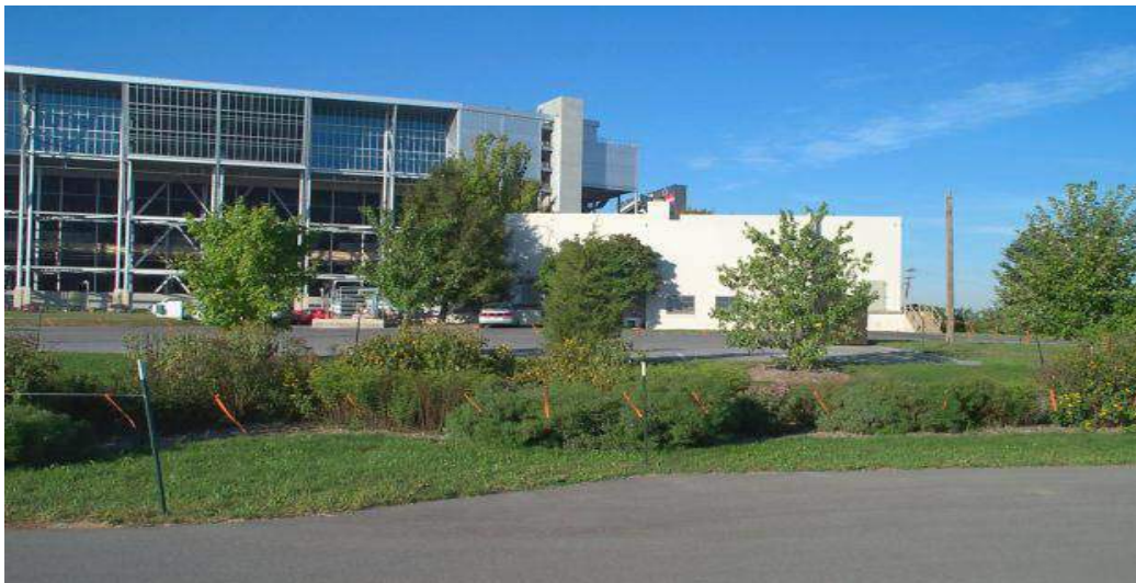
Figure 5.3.2-5. This landscaped area is underlain by an infiltration bed. The bed receives runoff from the upslope impervious areas.
