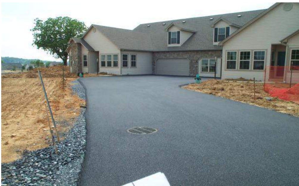
Figures 5.3.2-3a and b. Infiltration beds were incorporated into standard asphalt driveways in this suburban residential development. Standard asphalt was chosen for ease of maintenance and to prevent homeowners from inadvertently “seal coating” porous pavement. Roof leaders convey runoff directly into beds. The sumped catch basin serves to connect the bed to the storm sewer and may also collect driveway and surface runoff. The roof leaders from the house include cleanouts.
