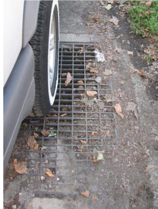
Figure 5.3.3-9. Lack of inlet maintenance can prevent water from entering an urban tree trench.
