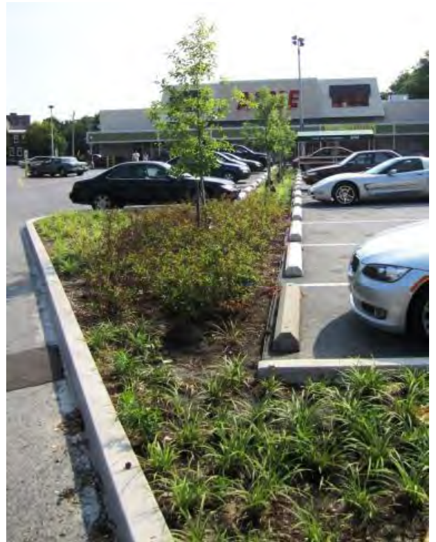
Figure 5.3.4-12. Edge conditions in a commercial parking lot allow for direct and unconcentrated surface flow into the adjacent bioretention area.
