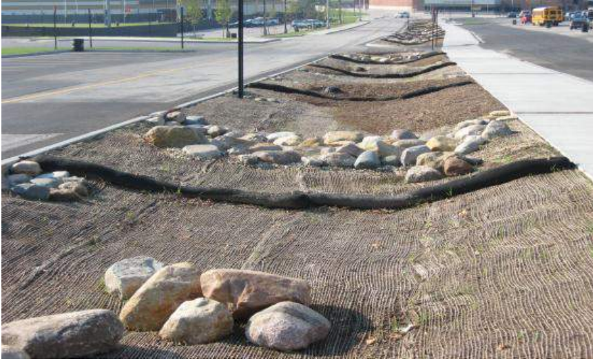
Figure 5.3.5-4. This vegetated swale on a slope includes stone check dams to slow runoff and earthen check dams to retain runoff.
