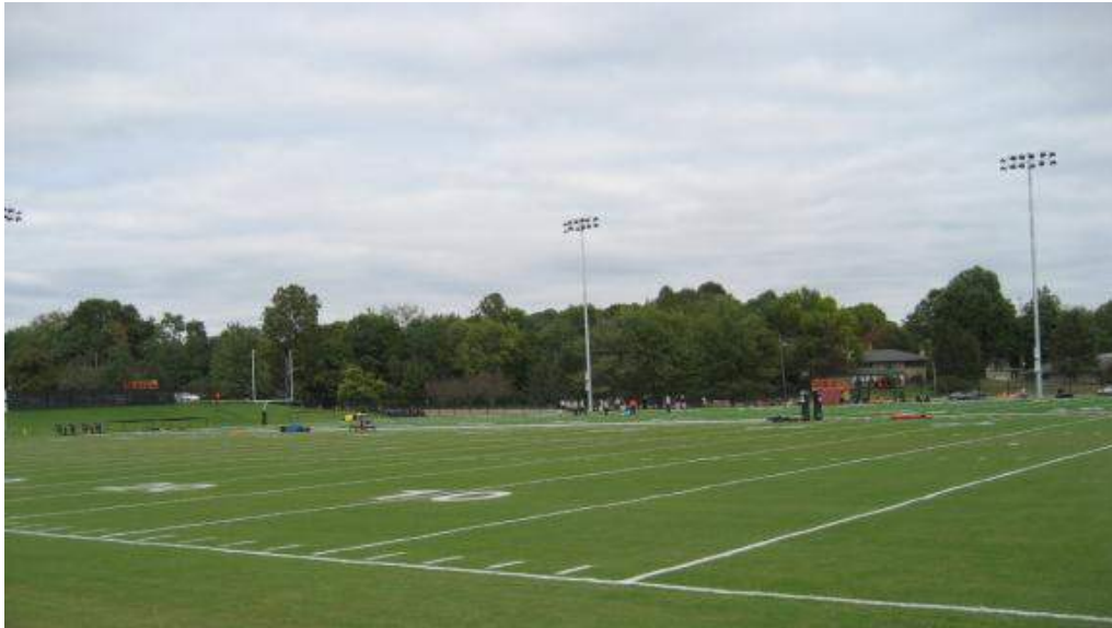
Figure 5.3.2-4. An infiltration bed beneath large athletic fields at Purdue University serves as a regional stormwater system for the campus. The two football practice fields are nearly 3 acres in area and capture runoff from the fields as well as nearly 10 acres of parking lots and roads. Runoff from parking lots and roads is pretreated with bioretention and vegetated swales before being discharged into the bed.
