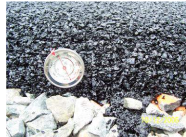
Figure 5.3.1-8. It is important that pervious pavement be placed at the correct temperature as determined by the drain-down test for the asphalt mix.
