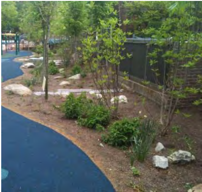
Figure 5.3.4-11. Edge conditions at a school allow for direct surface flow from the play area to the adjacent bioretention area.
