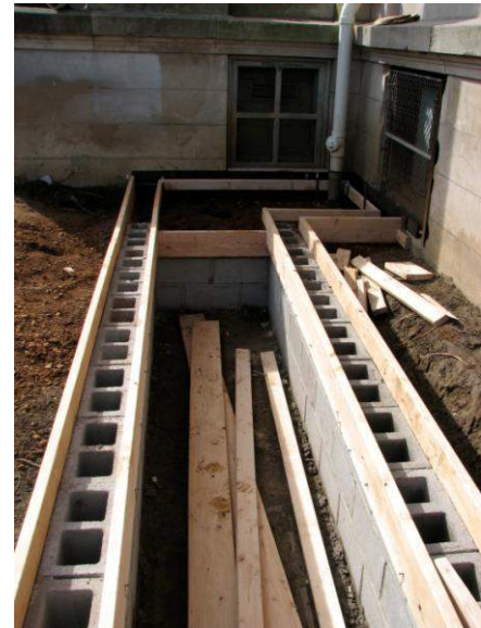
Figure 5.3.11-14. A stormwater planter box during construction. The sidewalls of the planter box are constructed once the final surface grade outside the box is met.
