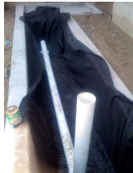
Figure 5.3.11-13. A waterproof liner is placed in the stormwater planter box to protect the adjacent building.
