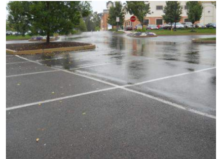
Figure 5.3.1-1. Rainfall drains directly through pervious asphalt pavement (left side of photo) but can be seen as runoff on standard impervious asphalt pavement (right side of photo).
