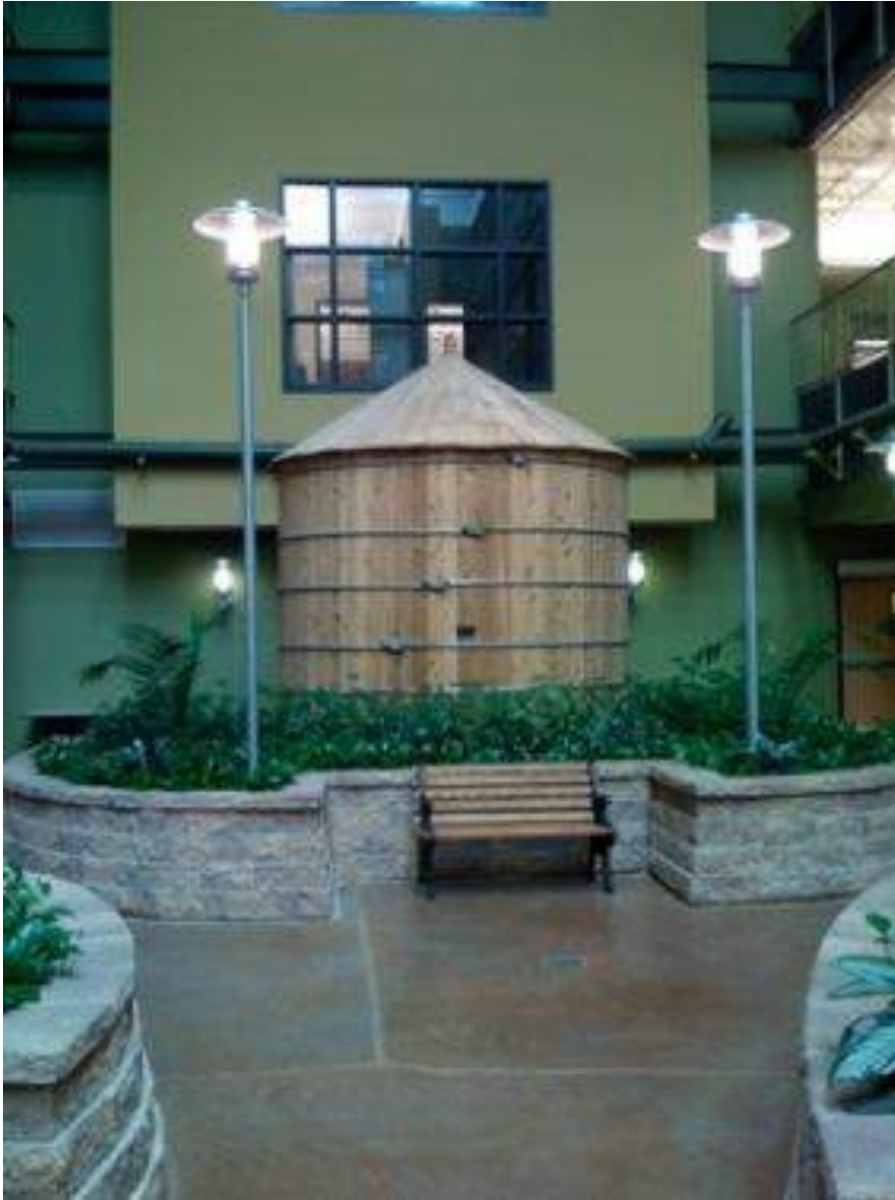
Figure 5.3.9-6. This cistern is located indoors. Roof runoff is captured for toilet flushing within the building.
