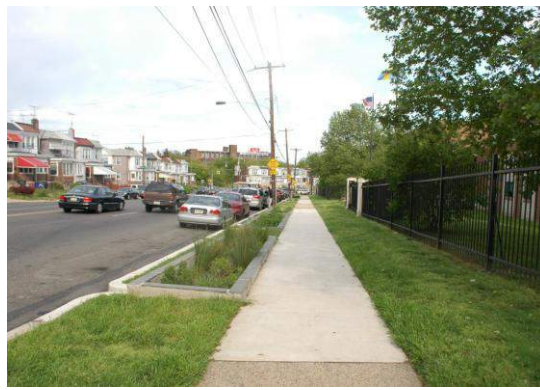
Figures 5.3.11-3a and b. This street was retrofitted to incorporate infiltration planter boxes within the right-of-way. Runoff enters the planter boxes through curb cuts.
