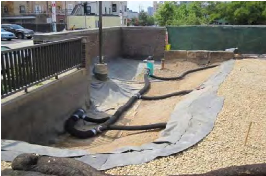
Figure 5.3.4-22. Installation of distribution pipes in bioretention area.
