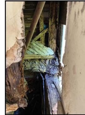
Photos #7 through #10 - Framing Damage
