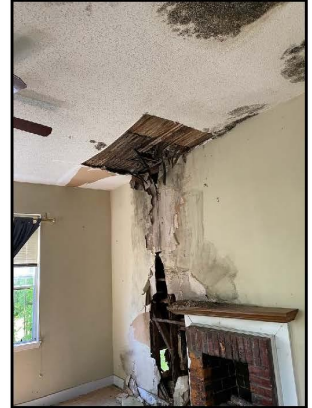
Photos #7 through #10 - Framing Damage
