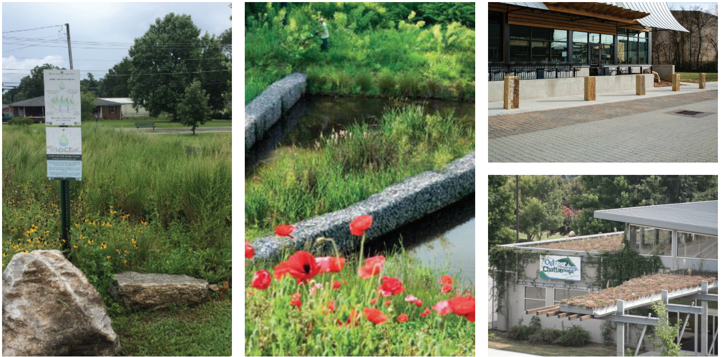
Examples of Green Stormwater Infrastructure projects in Chattanooga. Clockwise from top right: pervious pavers on Johnson Street in front of the Flying Squirrel; green roof at Outdoor Chattanooga; wetland restoration at Renaissance Park; and bioretention planting at John A. Patten Recreation Center.
