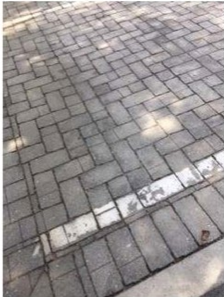
BMP Previous Pavement
