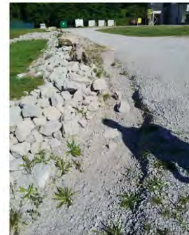
BEFORE MAINTENANCE: Gravel has washed out at the base of the rip rap filter dam. Sediment and weeds have accumulated and need to be removed.
