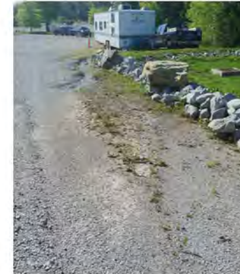
BEFORE MAINTENANCE: Gravel has washed out at the base of the rip rap filter dam. Sediment and weeds have accumulated and need to be removed.
