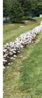
AFTER MAINTENANCE: clippings
