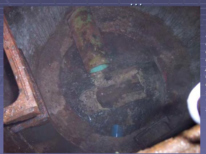
FOG impact may be immediately downstream of FSE or it may be 200+ feet downstream depending on slope of sewer, temperature of wastewater and surfactant content.
