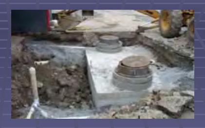
Grease Trap or "Inside, under-the-sink units", "floor traps", and "outdoor floor traps"
