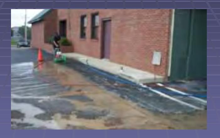
Replacement of sewer line outside a food service establishment due to FOG and soap film buildup
