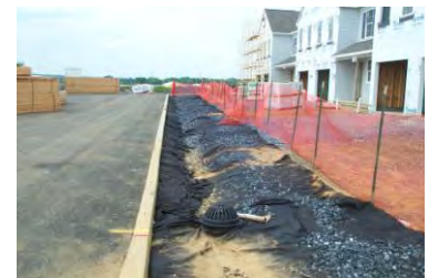
Figure 5.3.1-16. Extending the geotextile over the stone bed during construction of this pervious concrete sidewalk prevents sediment from entering the bed. In this example, the stone bed is wider than the sidewalk. It is designed to manage street runoff (from left) after treatment through a vegetated swale. Runoff sheet flows into the swale over the curb after construction of the final pavement course.
