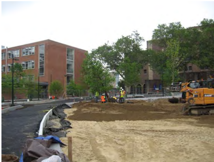
Figure 5.4.3-6. Designed soil layers being installed.
