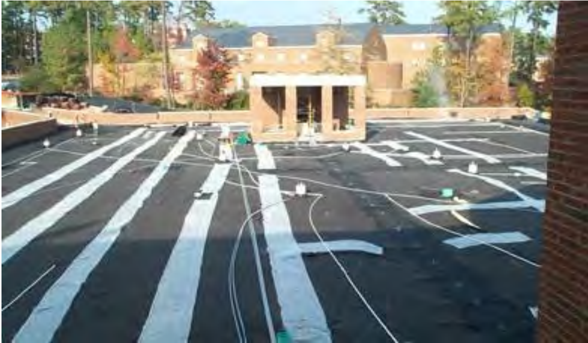
Figure 5.3.8-10. Geotextile and root protection.
