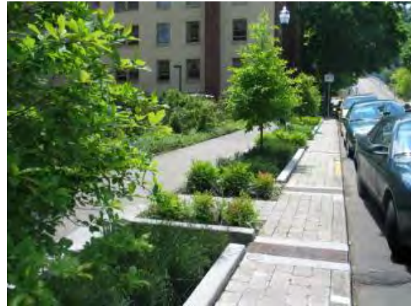
Figure 5.2.2-2. In densely urban areas—on streets, plazas, side yards, parking areas, etc.—drainage can be reinterpreted and integrated as a formal design with formal and ornamental plantings into the site amenities offered.
