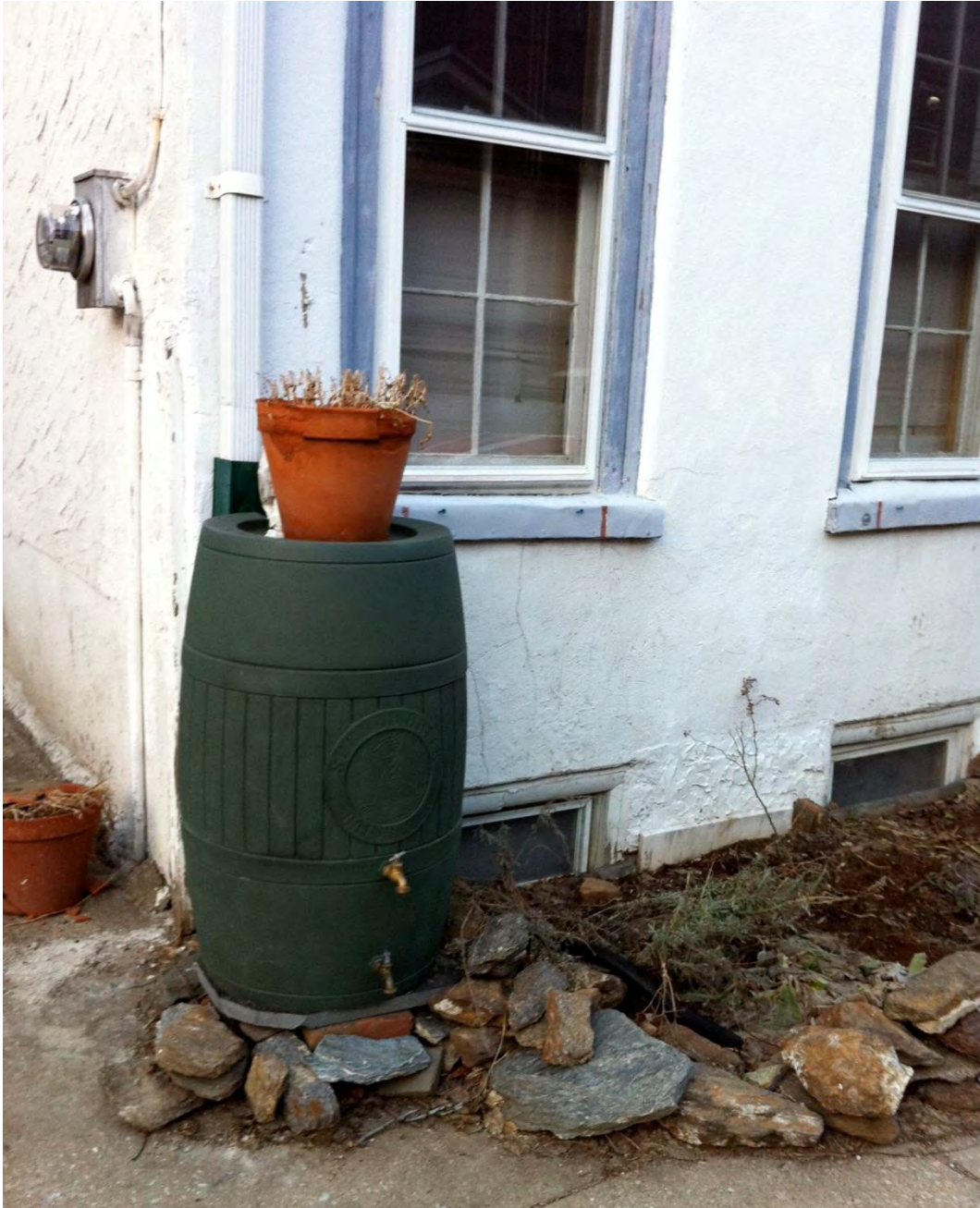
Figure 5.3.9-3. Rain barrels generally do not capture very large amounts of runoff, but are useful for increasing public awareness of stormwater issues.
