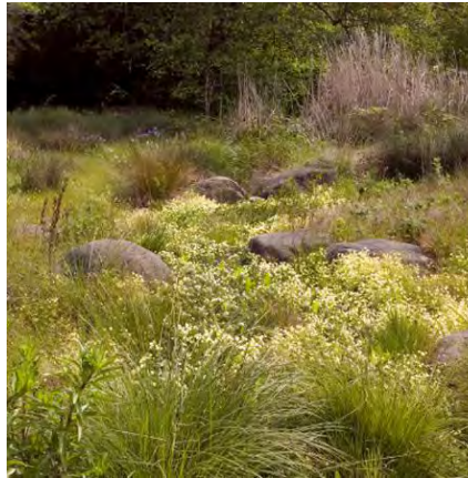
Figure 5.4.1-10. Vegetated swale – note meanders, rocks, grasses, etc. More pleasing to the eye than a straight swale, but still conveys stormwater and has more water quality functions.
