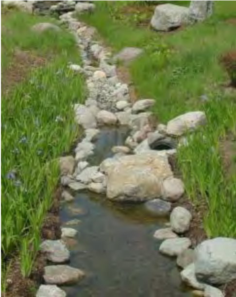
Figure 5.2.2-5. Stone reinforced swale.
