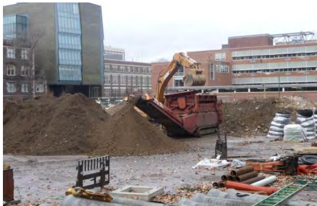
Figure 5.4.3-9. Urban soils being salvaged and mixed onsite.
