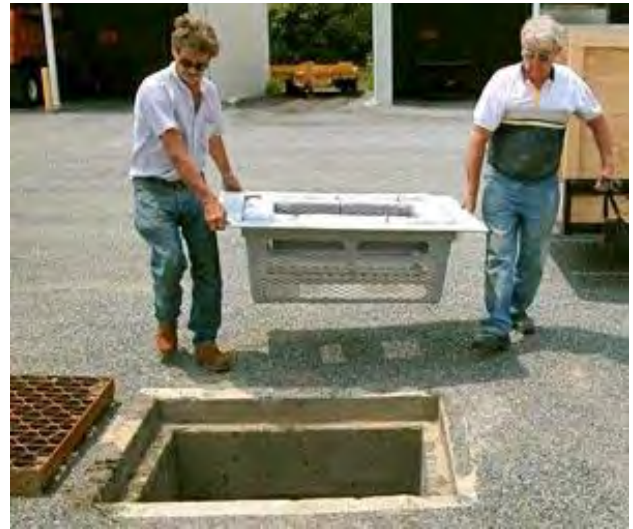
Figure 5.3.2-11. Water quality inserts can be used to reduce sediment and prevent trash from entering a stormwater infiltration bed. Water quality inserts require regular maintenance. ( http://www.gaelwolf2.com/dnrec/trib_times_2004_4_catch_basin_inserts.htm , Aug. 24, 2012)
