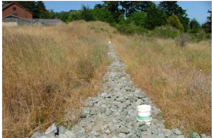
5.2.1.2-3. Level spreader along contour of slope.
