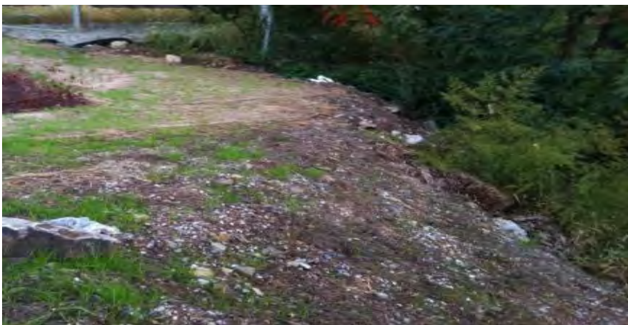
Figure 5.2.1.1-6. Example of abrupt transition between new and existing grade
