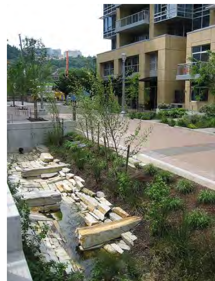
Figure 5.4.1.1-13. Energy dissipation at outfall structure.
