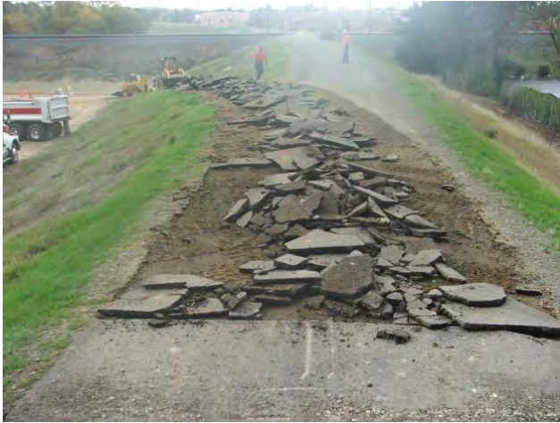
Figure 5.4.2.1-18. Pavement removal.
