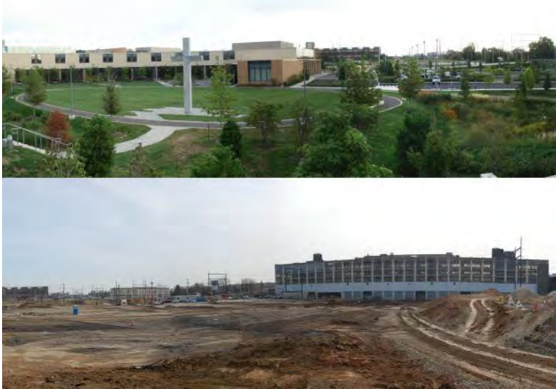
Figure 6-3. This Salvation Army facility is located on a brownfield site and applied better stormwater management practices.
