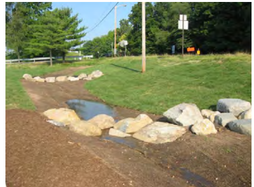
Figure 5.4.1.1-7. Vegetated swale retrofit with meadow seeding and check dams along roadside.
