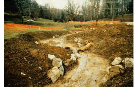
Figure 5.4.1-5. Recreating a meander within a channel, note boulders and curves, and that the right side is higher than the left, which has area for overflow if the water “jumps” the channel banks.
