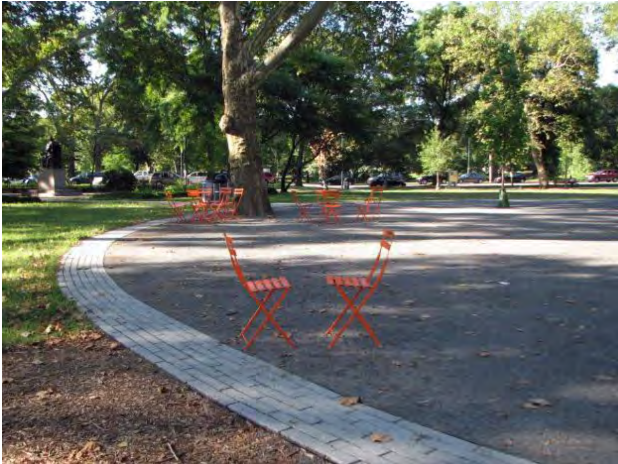
Figure 5.3.2-6. This urban park plaza is built above an infiltration bed that completely underlies the plaza. Runoff is both piped into the bed from adjacent areas and is able to enter the bed through the porous pavers around the perimeter of the plaza.
