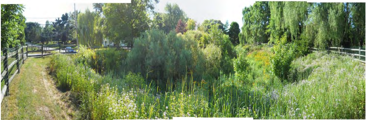
Figures 5.3.13 -1a and b. This detention basin in a residential neighborhood was retrofit to become a naturalized detention basin.
