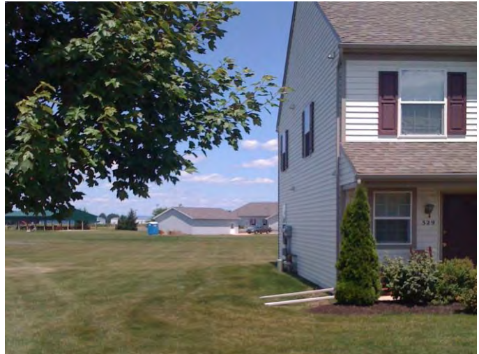
Figure 5.3.10-1. Roof leaders from a residence sheet flow across turf and, eventually, to a meadow area, which filters and absorbs stormwater runoff.
