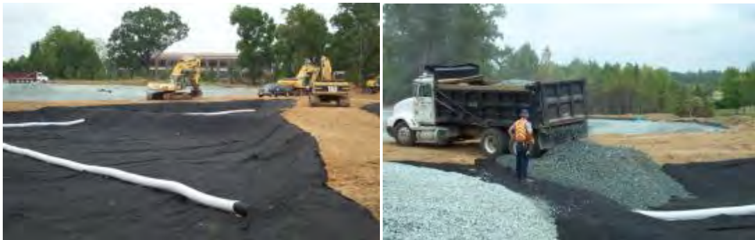
Figures 5.3.1-20a and b. Geotextile and perforated distribution pipes are placed on an uncompacted subgrade, and stone is placed without compacting the bed bottom. Distribution pipes can be designed to extend through berms within the bed.
