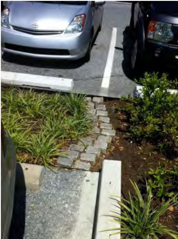
Figure 5.3.4-8. Cobbles in the bioretention area allow for easy and safe pedestrian crossing without disturbing soils and vegetation.
