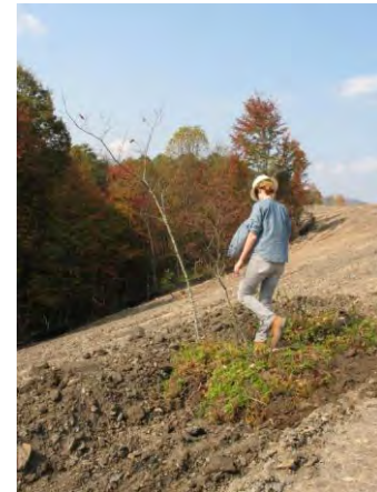
Figure 5.2.4.2-8. Meadow sod placement – foot tamping.
