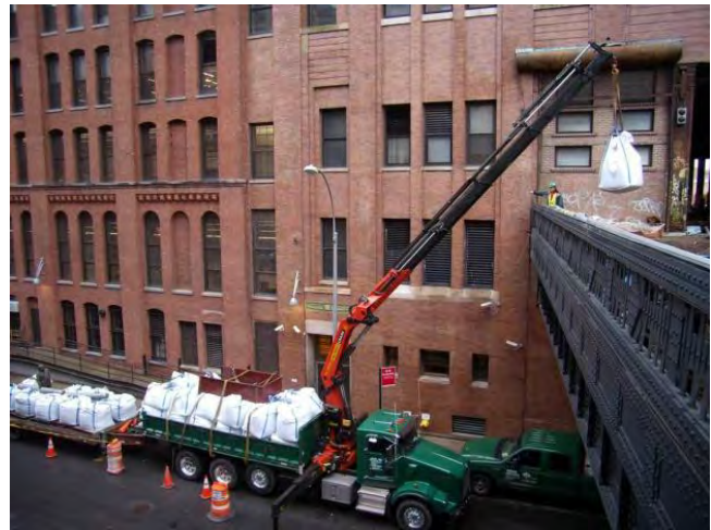
Figure 5.4.3-4. Soil being delivered to an elevated planting site.
