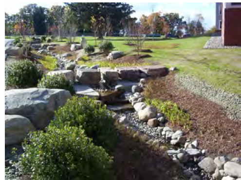
Figure 5.4.1.1-12. Naturalized swale with check dams and river-rock reinforced channel.
