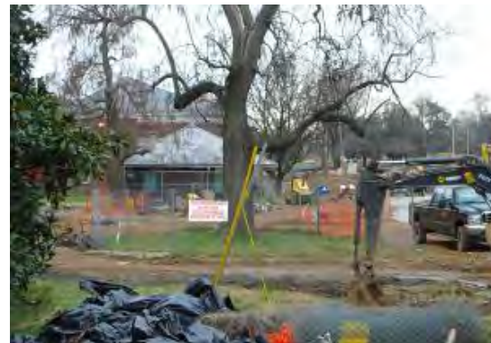
Figure 5.2.4.1-2. Tree protection fence with sign.
