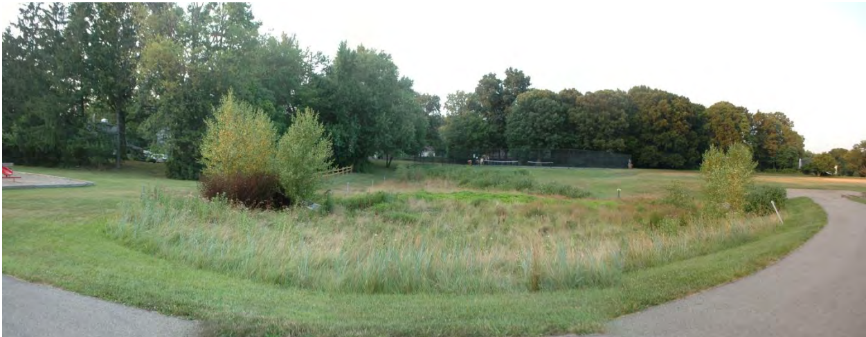
Figures 5.3.13-5a and b. The existing detention basin in this community park was modified to capture ½-inch rainfall events and to eliminate an erosive flow path condition.
