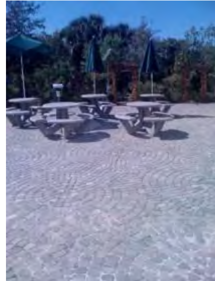
Figure 5.3.1-4. Pervious concrete pavers for terrace area. Pervious pavers are ideal for plaza and terrace areas.
