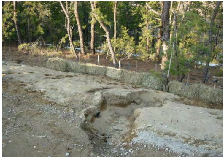
Figure 5.2.1-8. Soil protection at woodland edge.
