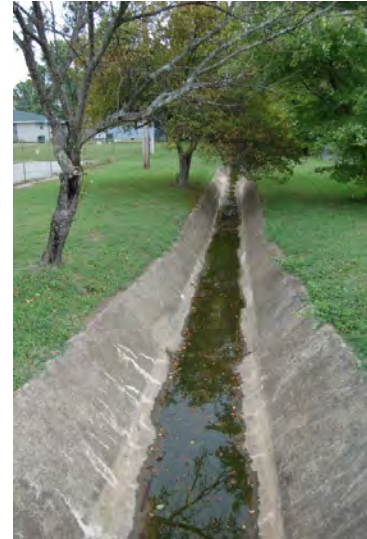
Figure 5.4.1.1-3. Concrete drainage channel in Chattanooga.
