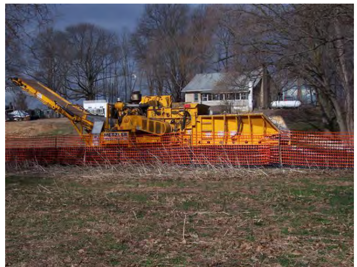
Figure 6-4. Unnecessary material storage and equipment movement can compact soils, resulting in more runoff after construction. Clearly limiting vehicle access to unpaved areas can improve soil conditions adjacent to roadways.
