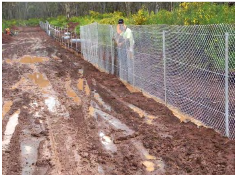
Figure 5.2.1-6. Construction site fencing protecting healthy soil under forest cover.
