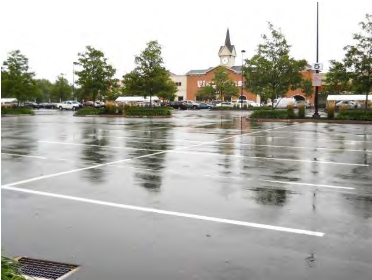
Figure 5.3.2-8. This supermarket parking lot required a level surface. Infiltration beds were placed at the native soil interface, beneath the fill material and parking lot.
