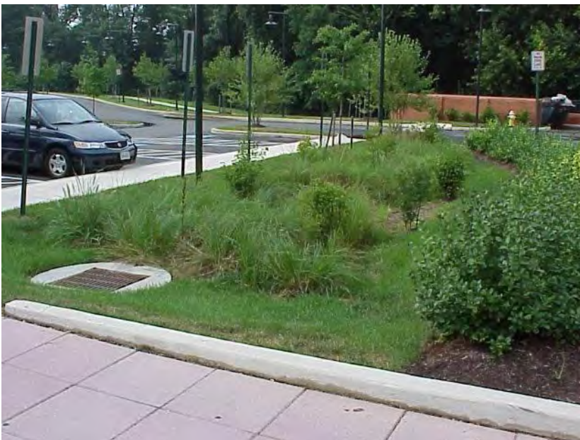
Figure 5.3.4-6. Commercial bioretention (rain garden) in parking lot.
