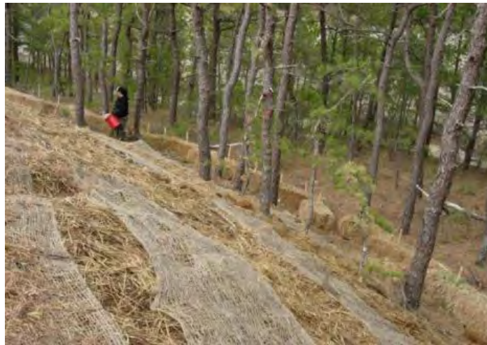
5.2.1.2-7. Steep slope erosion management installation.
