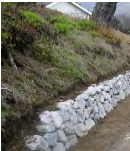
5.2.1.2-2. Steep slope stone wall.
