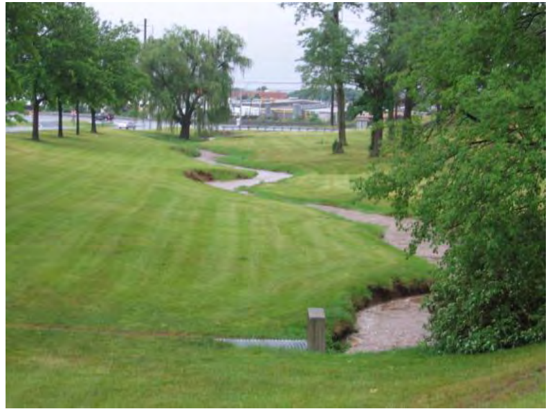
Figure 6-6. A stormwater pipe discharging roadway runoff directly into an urban stream during a rainfall event.
