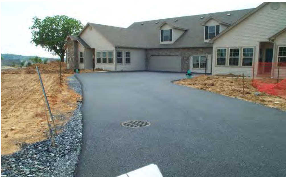
Figures 5.3.2-3a and b. Infiltration beds were incorporated into standard asphalt driveways in this suburban residential development. Standard asphalt was chosen for ease of maintenance and to prevent homeowners from inadvertently “seal coating” porous pavement. Roof leaders convey runoff directly into beds. The sumped catch basin serves to connect the bed to the storm sewer and may also collect driveway and surface runoff. The roof leaders from the house include cleanouts.
