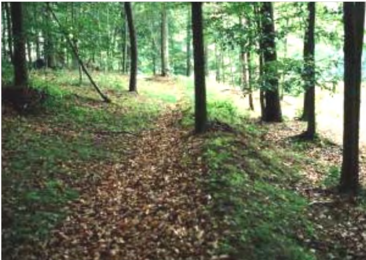
Figure 5.3.7-1. Infiltration berm constructed along the contour in a wooded area receives runoff from a large-lot residential area.
