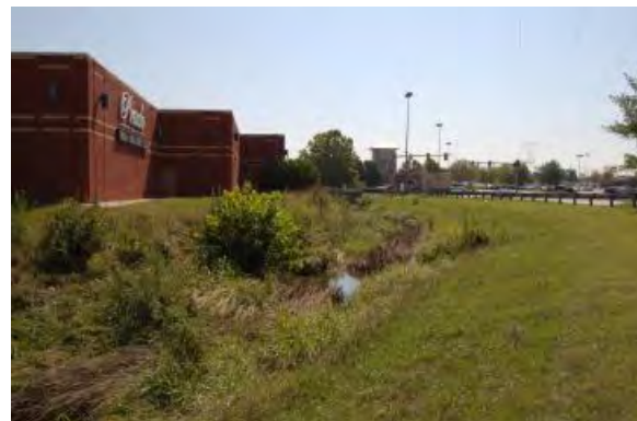
Figure 5.2.2-1. Open water channels for drainage (either natural or manmade) are still common within the Chattanooga region. In some cases, these channels have been straightened and lined with rip-rap or concrete. They can be found even on very urban sites, such as this one at the Hamilton Place Mall.
