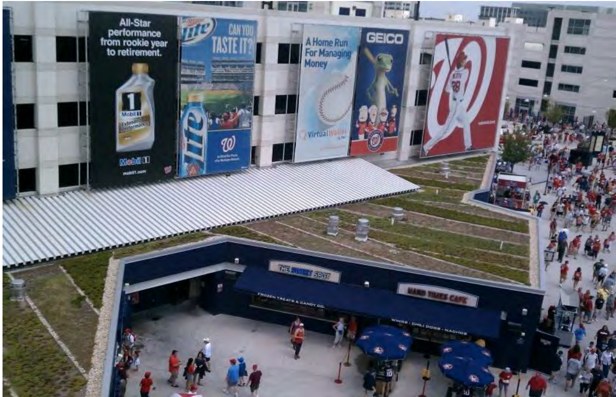
Figure 5.3.8-7. Green roof at a Washington Nationals Stadium.
