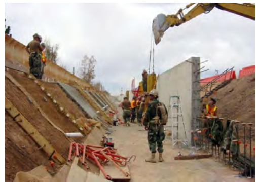
Figure 5.4.1.1-2. Concrete channel under construction.
