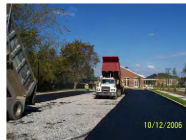
Figure 5.3.1-21: Although the subgrade is uncompacted to allow for infiltration, the stone bed is placed in layers and rolled to provide a suitable subbase for construction vehicles and future traffic loads.
