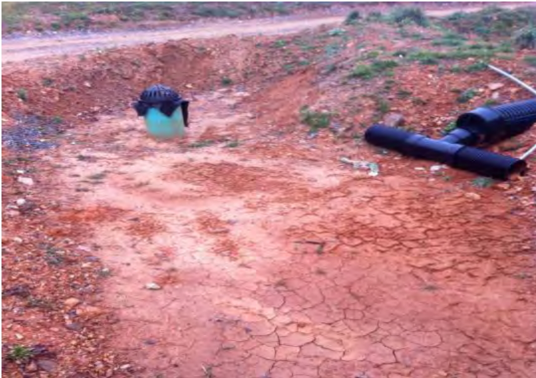
Figure 5.3.4-21. An underdrained bioretention area is used as a sediment trap during construction.
