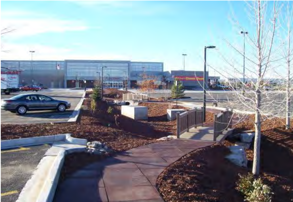
Figure 5.3.5-6. The parking lot vegetated swale at this commercial center is designed for pedestrian crossings.
