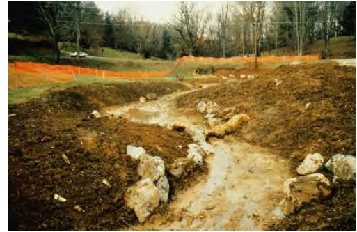
Figure 5.2.2-8. Channel design in construction.
