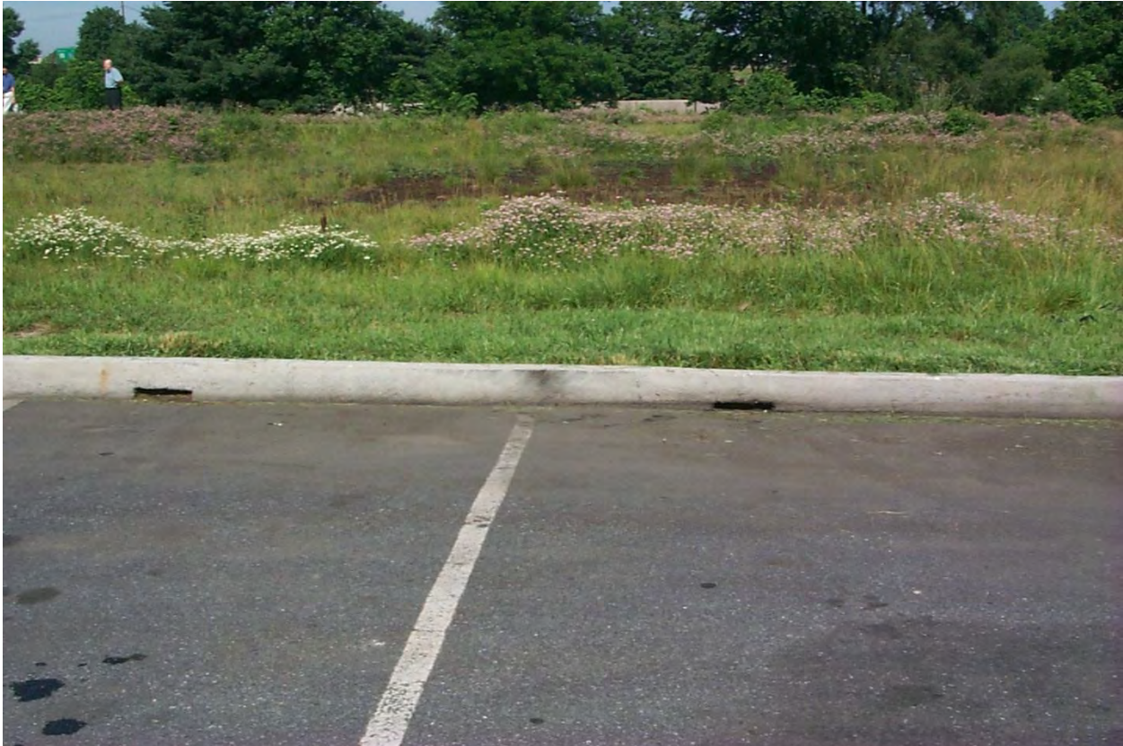
Figure 5.3.10-5. A parking lot is disconnected by directing flow through curb cuts to a vegetated area that includes a filter strip.
