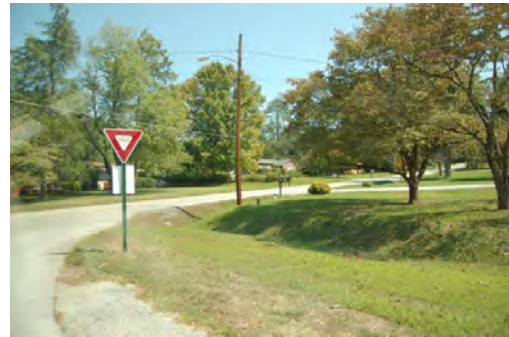
Figure 5.4.1.1-9. Drainage channel street side in residential area in Chattanooga, Tennessee.
