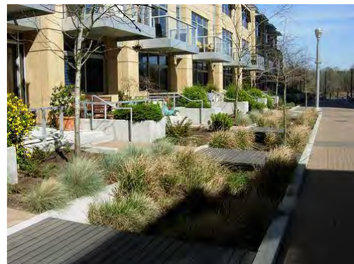
Figure 5.4.1.1-10. Vegetated swale in apartment complex in Portland, Oregon.
