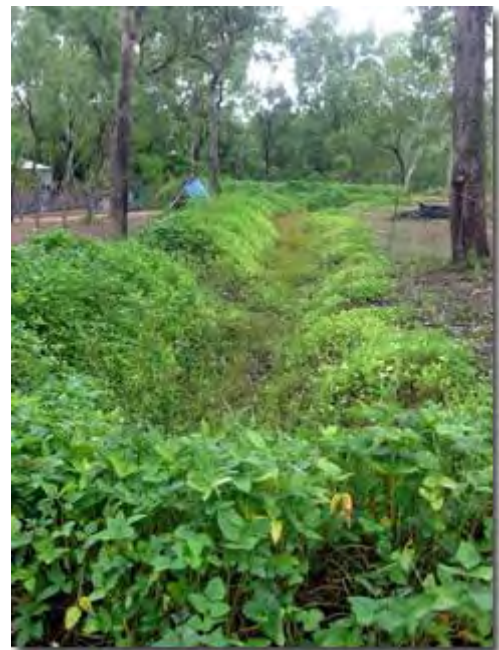
Figure 5.2.2-3. Existing drainage corridors and their buffering vegetation can be expressed as a rural drainage ditch.
