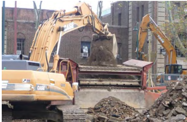
Figure 5.4.3-8. Urban soils being salvaged/sorted and debris being removed.
