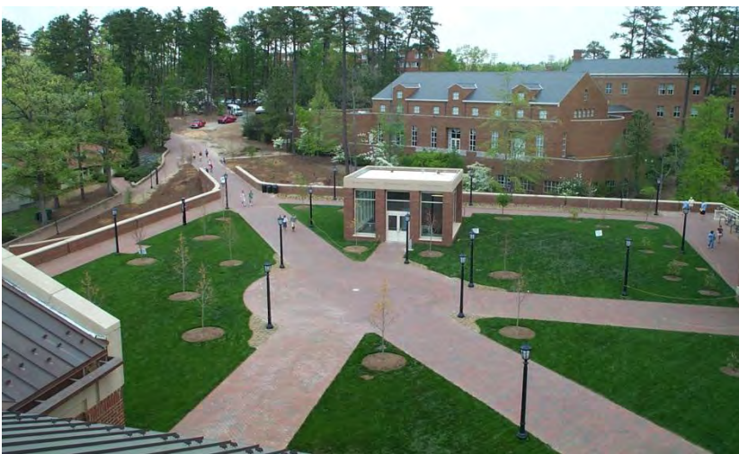
Figure 5.3.8-6. Extensive green roof plaza atop a parking garage at UNC Chapel Hill.
