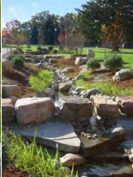
Figure 5.2.2-6. Reinforced swale bottom and check dam.
