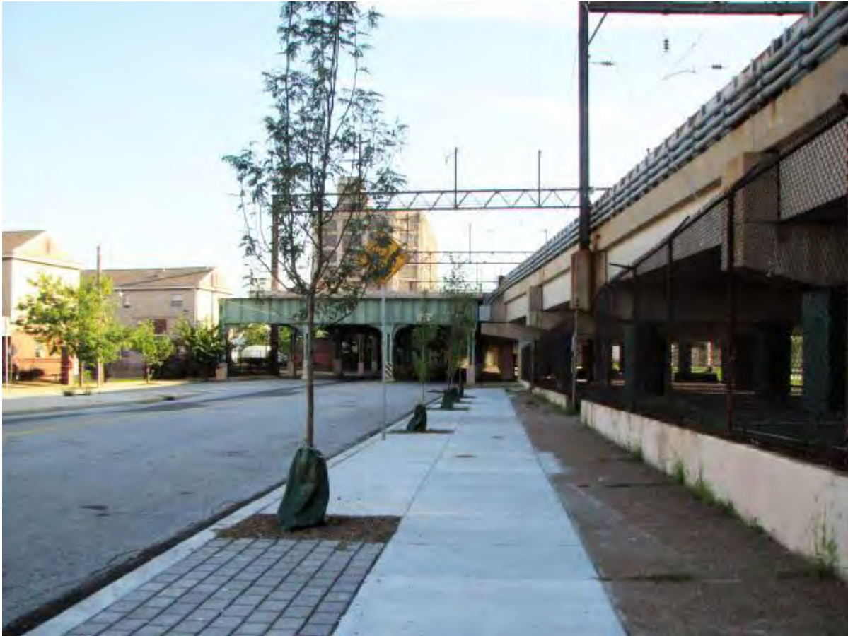
Figure 5.3.3-5. Tree trenches capture street runoff, via curb inlets, and improve urban greening and streetscapes, especially in ultra-urban locations.
