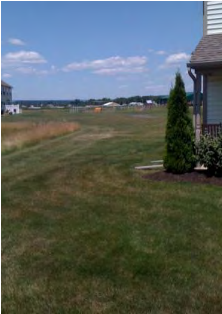
Figure 5.3.6-4. Roof leaders convey runoff to a vegetated filter strip in a residential neighborhood.
