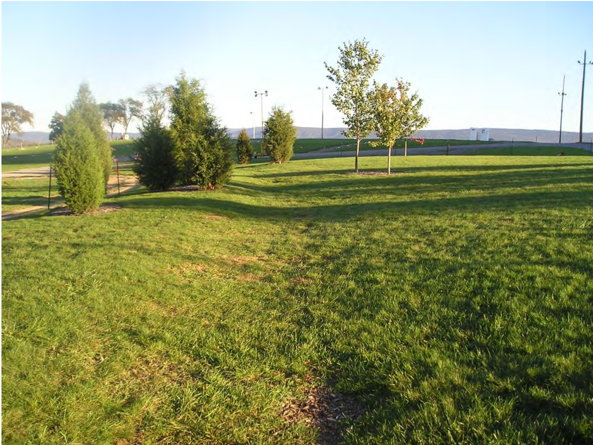
Figure 5.3.7-2. This berm is combined with an infiltration trench (BMP 5.3.3) to capture runoff from a grassed overflow parking area.
