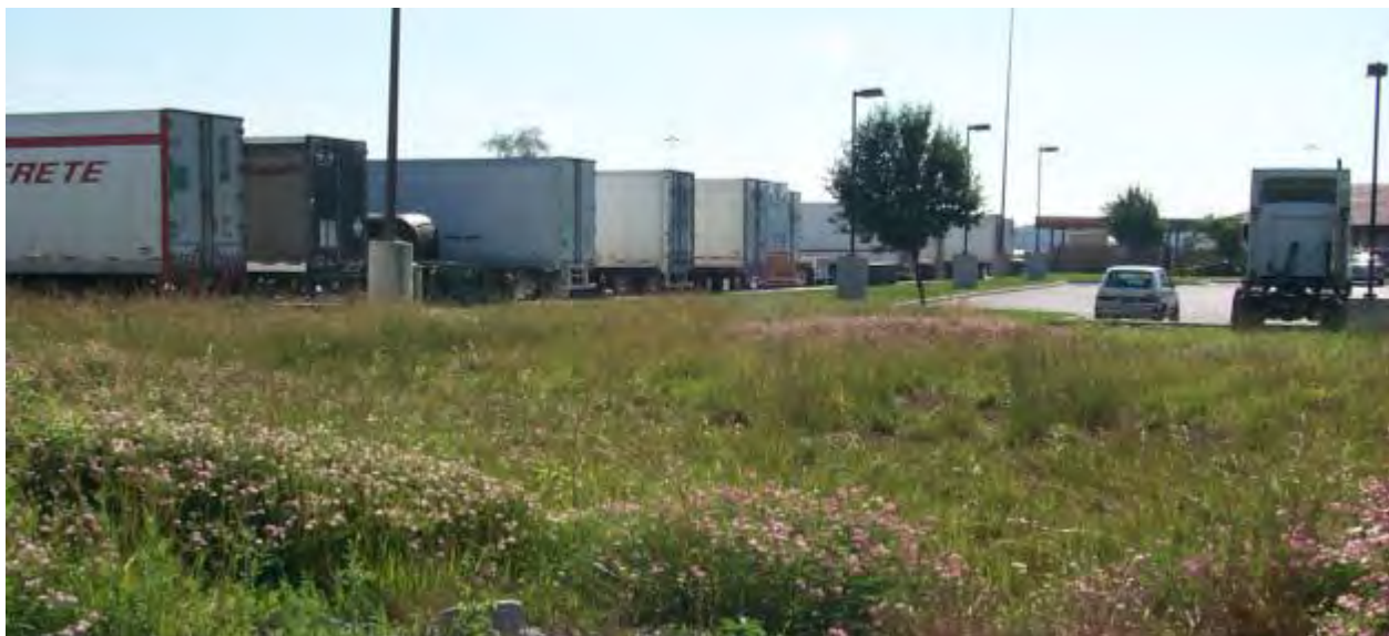
Figure 5.3.6-5. The parking lots at this truck stop discharge to filter strips before being conveyed to bioretention and infiltration areas.
