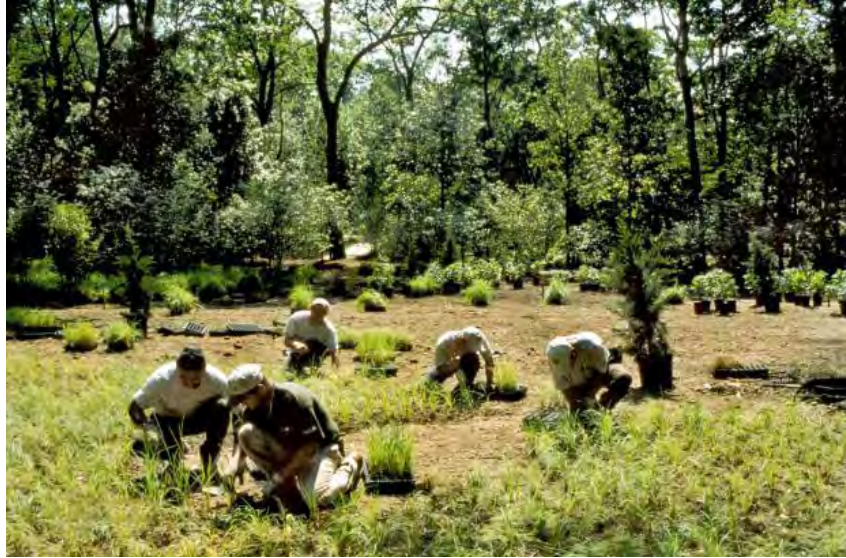
Figure 5.4.2.1-11. Meadow plugs being installed.
