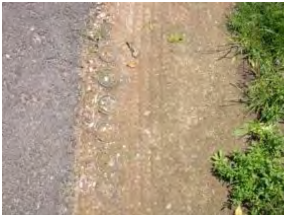
Figure 5.3.1-7-e. Reinforced Turf or Gravel
