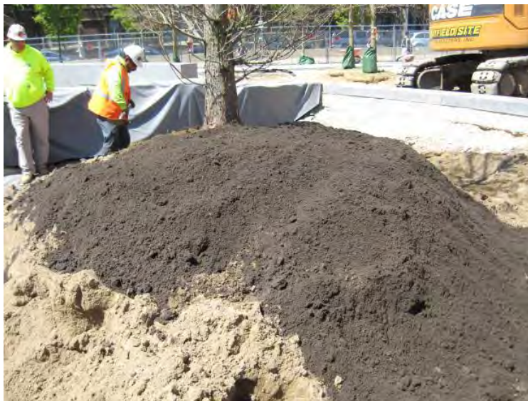
Figure 5.4.3-7. Close-up of designed soil layers.
