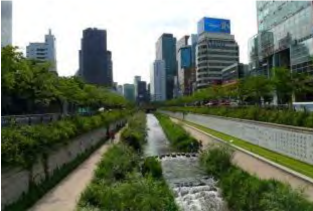
Figure 5.2.3-5. Urban Example – Cheonggyecheon River Restoration Project.
