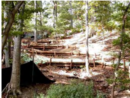
Figure 5.4.1-7. Log check dam installed.
