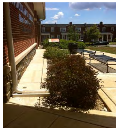
Figure 5.3.11-5. Flow-through stormwater planter boxes adjacent to this library receive roof runoff and provide plantings within the hardscape seating area. Overflow from these planter boxes is directed to a bioretention area (right side of photo). River cobbles (not shown) were added to eliminate any tripping hazard in a high-use area by reducing the depth of the planter box edge to the finished surface.
