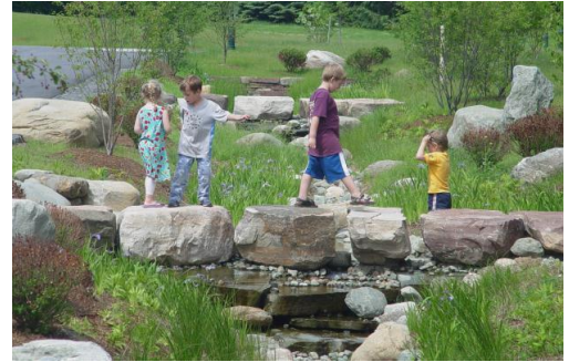
Figure 5.4.1.1-6. Vegetated swale with check dams in a residential neighborhood.
