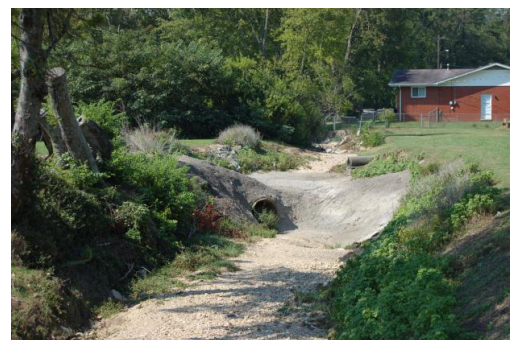
Figure 5.4.1.1-8. Drainage channel running behind a residential area in Chattanooga, Tennessee.
