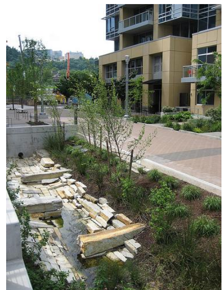
Figure 5.4.1.1-13. Energy dissipation at outfall structure.
