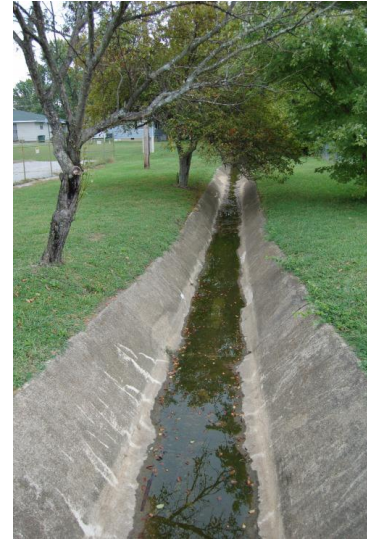
Figure 5.4.1.1-3. Concrete drainage channel in Chattanooga.
