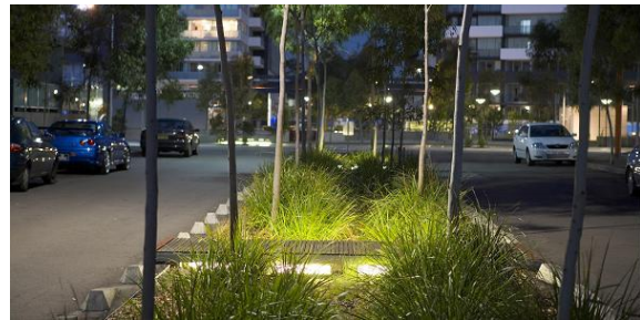
Figure 5.4.1.1-4. Highly urbanized, vegetated drainage swale.
