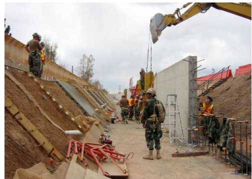
Figure 5.4.1.1-2. Concrete channel under construction.
