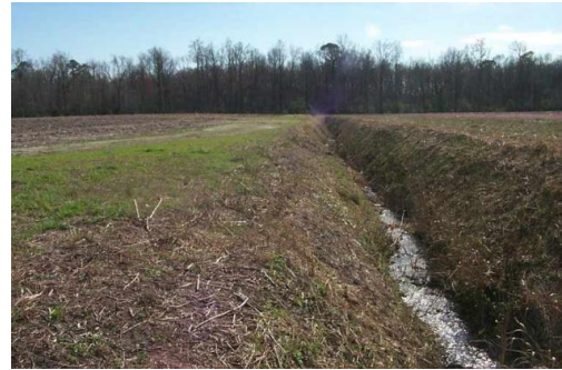
Figure 5.4.1.1-1. Typical farm channel.
