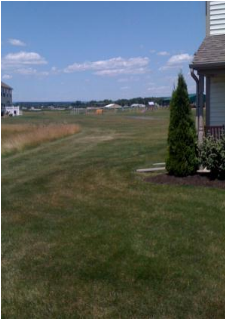
Figure 5.3.6-4. Roof leaders convey runoff to a vegetated filter strip in a residential neighborhood.
