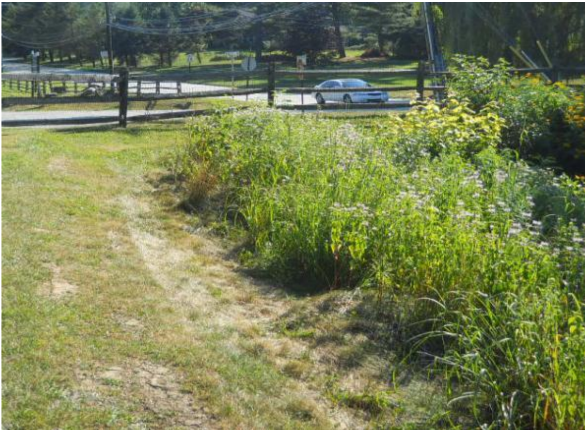
Figure 5.3.6-1. A meadow grass filter strip (long grass in the center of the image) provides a water quality buffer between a residential neighborhood and naturalized basin (far right).
