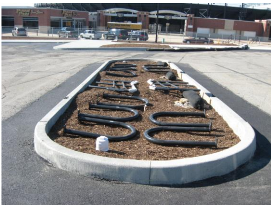
Figure 5.3.11-4. Infiltration planter box within a parking lot, during construction. Water will enter through curb cuts, which are closed during construction. Note that the asphalt around the planter box was milled and repaved, allowing it to drain to the curb cuts following construction.
